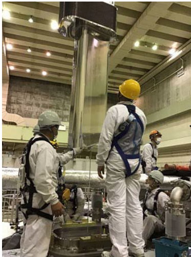
Installing the port into the tokamak (P-14)
