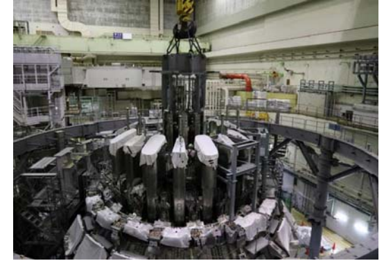
CS cannot be accessed for conventional repair in situ
