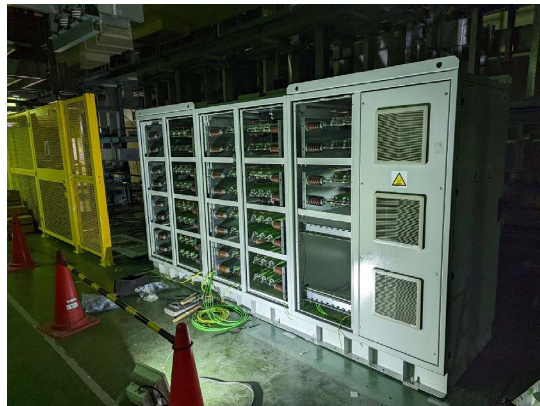
New "R2" grounding resistors under installation
