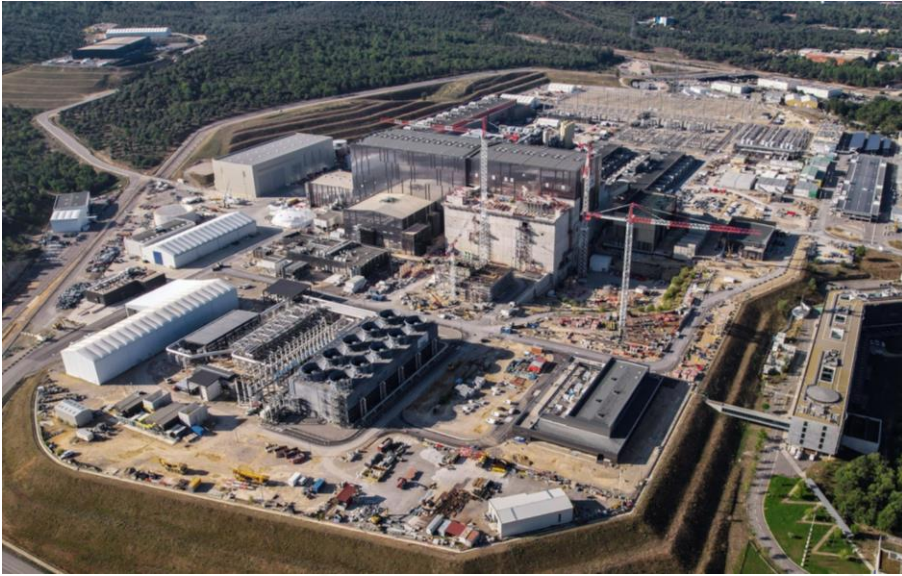
ITER site, September 2023 . ©ITER
