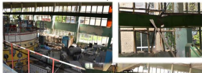
Stellarator hall inside Facilities still alive!
