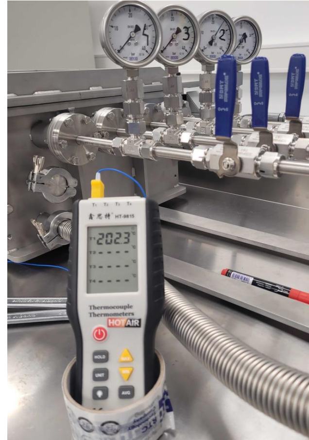
Hot leak test at 200 C 25 bar
