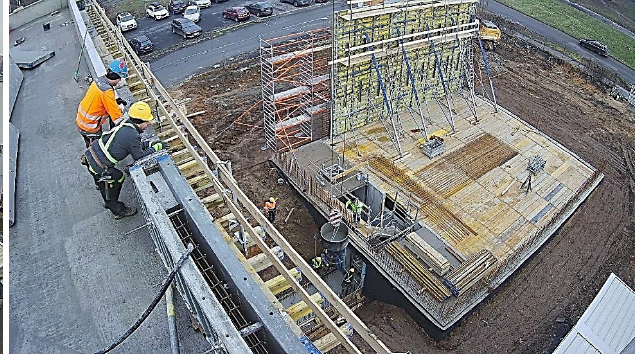
Basement for two fly-wheel generators
