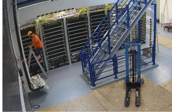
Installation of IGBT power supplies for PF coils
