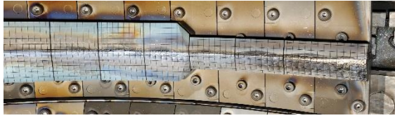
Melting along dump plate due to disruptions
