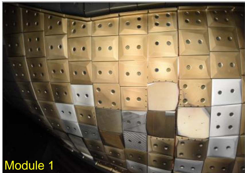
IPP_D_2KLQUC: Photo documentation of PV after MP2.2
